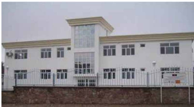
Hospital Provincial de Qala-i-Naw
